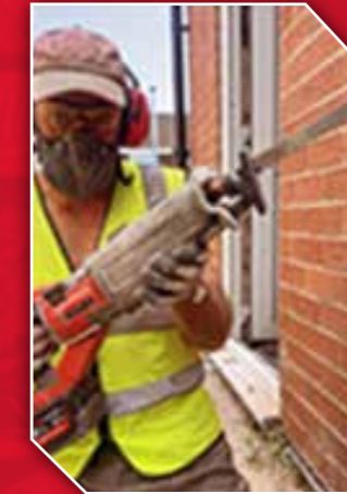
BRICKLAYING WITH STEVE & ALEX CONSTRUCTION YOUTUBE & INSTAGRAM
